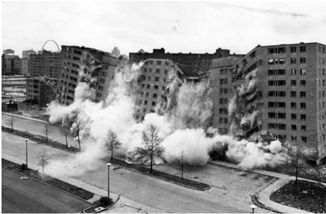
Pruitt-Igoe demolition, April 1972
